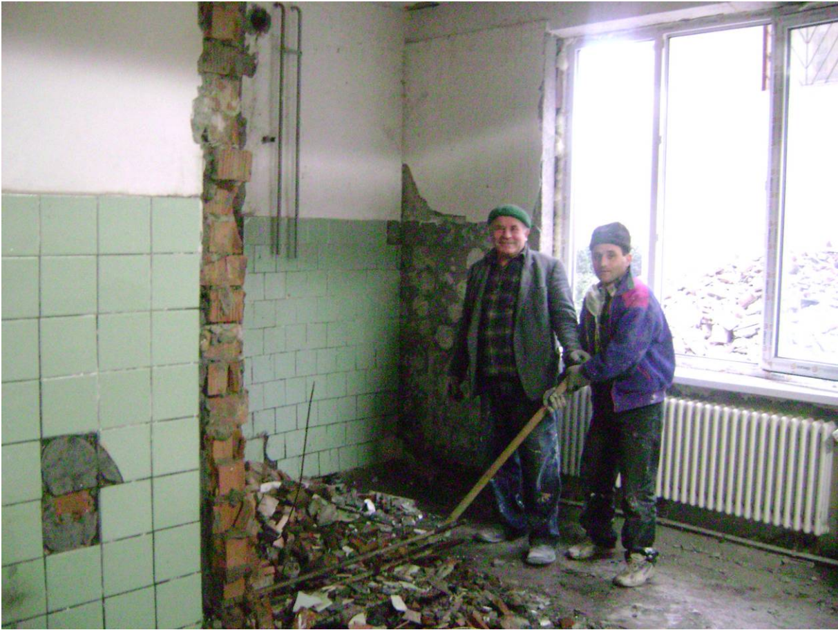
Figure 4. Start of the renovation of the basement in December 2009
